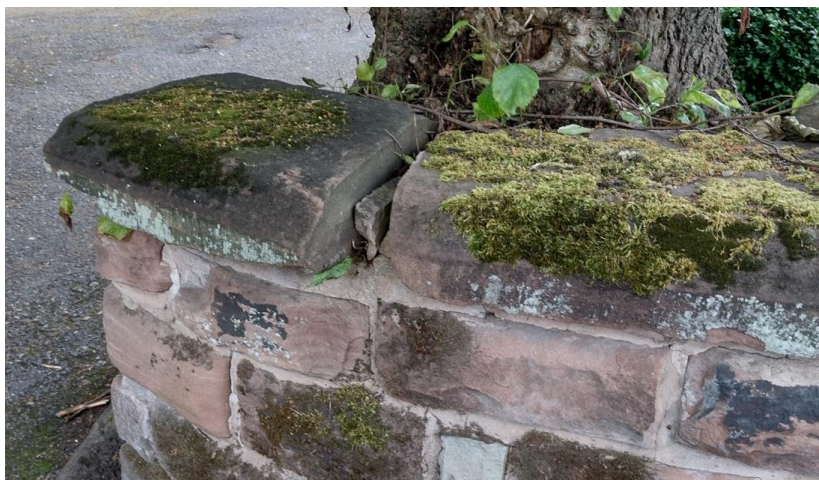
Image 2: Photos of base of protected trees, site access and boundary wall – taken 13 th July 2023.
